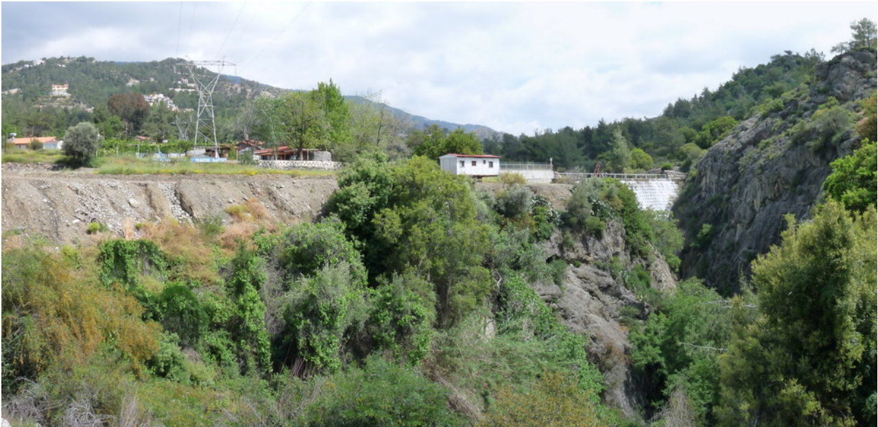
Figure 7 - TRIMIKLINI : Kouris valley seen from the B8 road bridge. At the background TRIMIKLINI Dam. The earth fill embankment for the gas station is on the left (right bank) – 180° photomontage.
