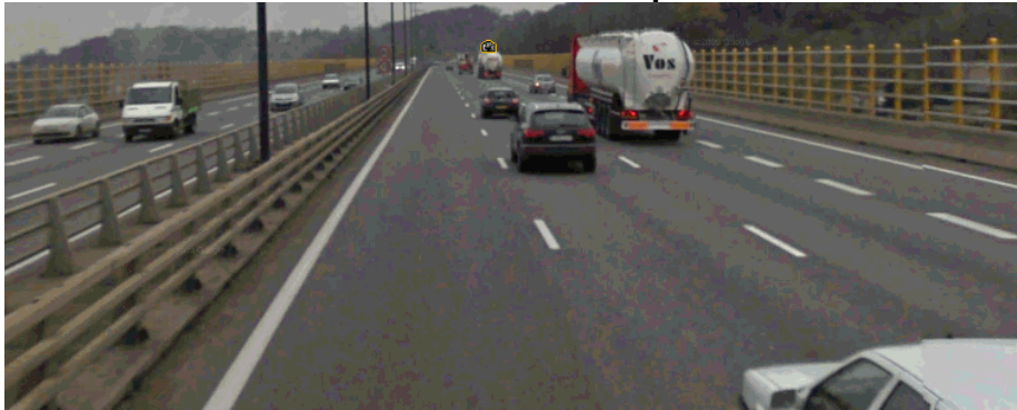
Exemple of strong crash barriers installed on a highway bridge which passes over a water body used for drinking water alimentation (France – Lyon).
