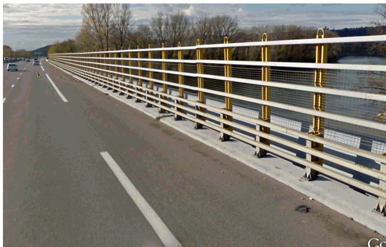
Idem, with a net to avoid the throwing of objects into the river.
