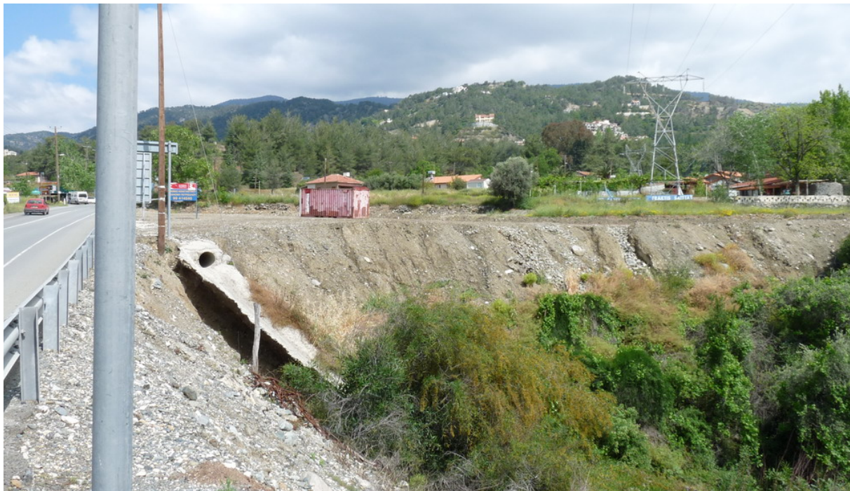
Figure 8 – TRIMIKLINI : The earth fill embankment for the gas station seen from the B8 road bridge showing already significant erosion of the edge (concrete ditch earth support disappeared)
