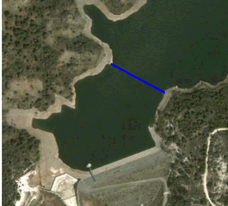
Figure 2 - Arminou, buoy line protection (blue line)
