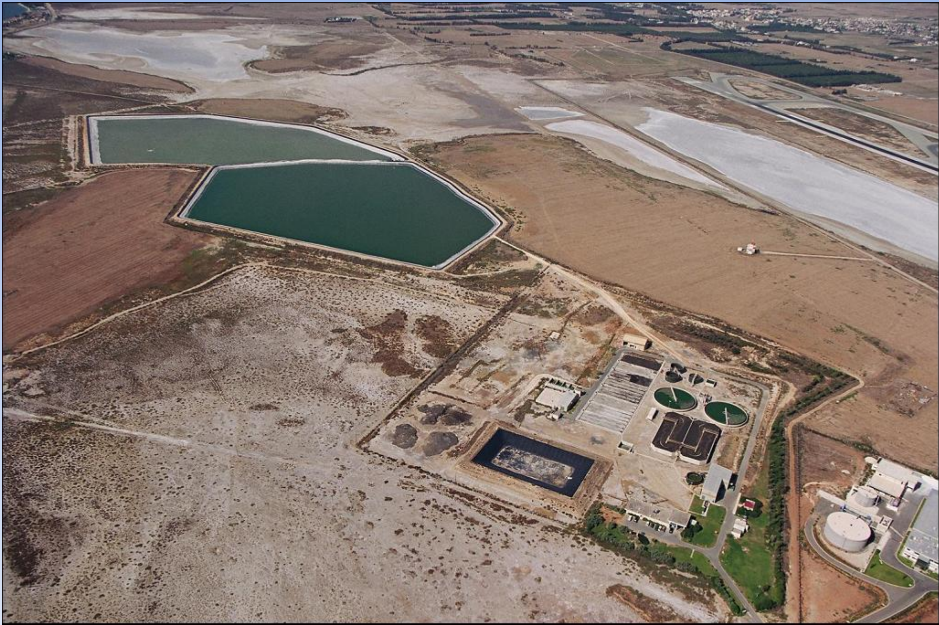
LARNACA WASTEWATER TREATMENT PLANT, SBL - 18,000 m 3 /day
