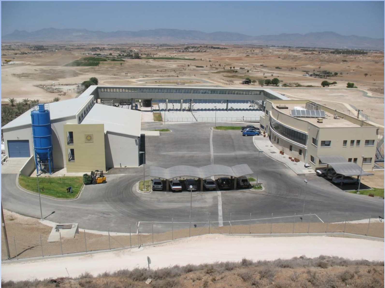
ANTHOUPOLIS WASTEWATER TREATMENT PLANT, SBN 13,000 m 3 /day
